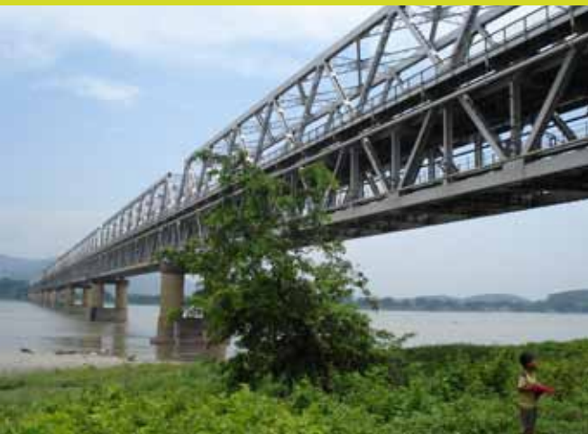
We provided construction supervision services for the bridge across Brahmaputra River near Guwahati in the state of Assam. This is part of a larger project which includes the bridge and approaches stretching for a total length of 5000m.
