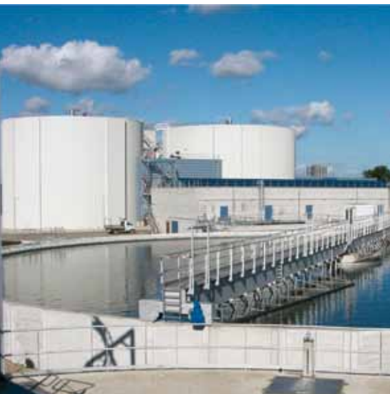
As technical advisor to the lead arrangers, Mott MacDonald provided support throughout the development of the new 31,800 m 3 /hour Harnaschpolder wastewater treatment plant in the Netherlands.
