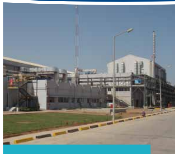
We were appointed as the EPCM consultant for the Greenfield offset printing ink manufacturing facility in the state of Gujarat.
